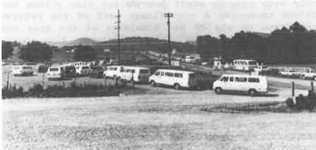
Figure 3. Quitting time at Hartsville construction site.
