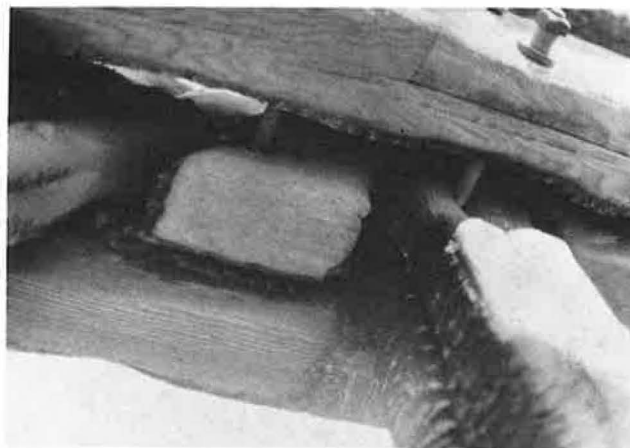
Figure 8. Typical joint destruction.
