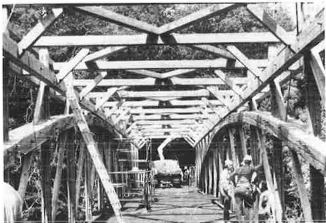
Figure 12. Installation of top lateral system.
