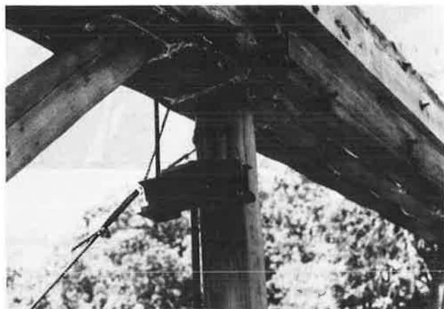
Figure 11. Auxiliary hanger system at middle verticals.
