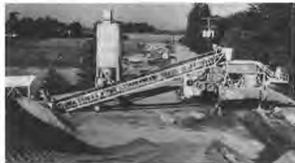
Figure 2. Batch and mix plant for cement-stabilized base materials.
