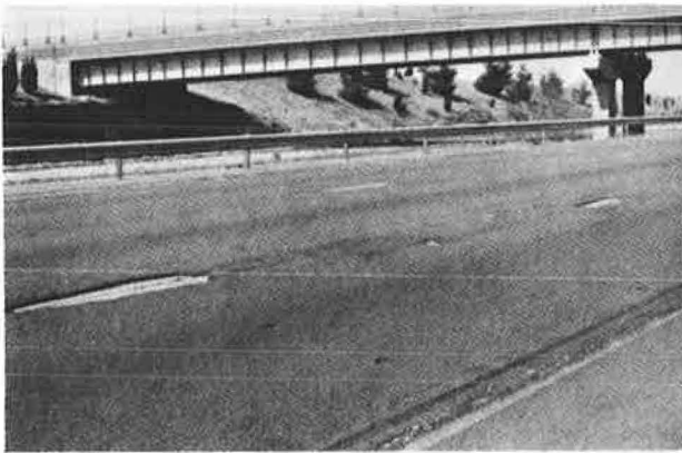
Figure 9. Overview of portion of test section 3N.
