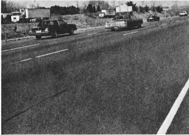
Figure 3. Gouge marks from hard object in surface of open-graded material (southbound, control section).
