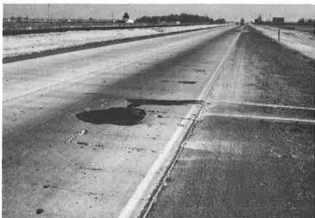
Figure 20. Pumping associated with continuously reinforced concrete pavement.
