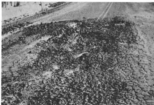
Figure 2. Spring breakup due to poor subsurface drainage.
