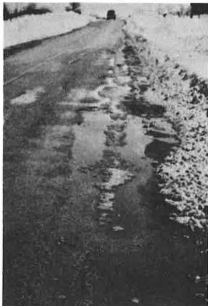
Figure 1. Snowmelt trapped by plowed snowbanks.
