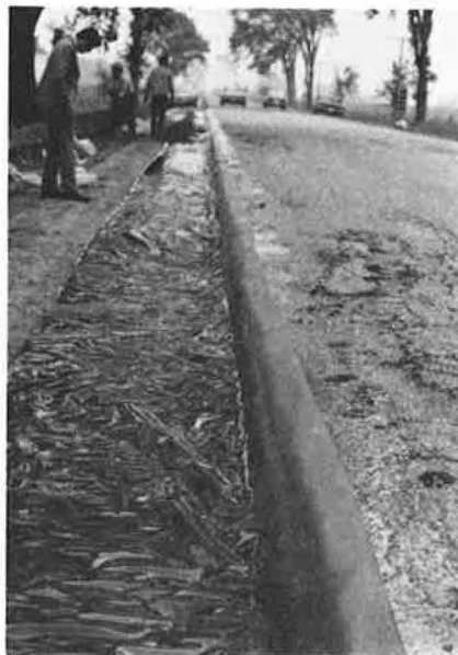
Figure 3. Plastic edge skirts in gravel shoulder.
