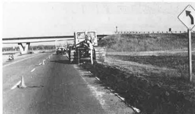
Figure 5. Installing plastic pipe subdrains by using trenchless plow.
