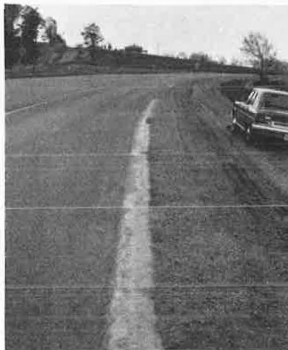
Figure 11. Primed gravel shoulder three years after application.
