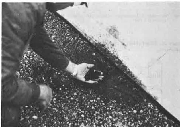
Figure 21. BAM pumped from beneath continuously reinforced concrete pavement.
