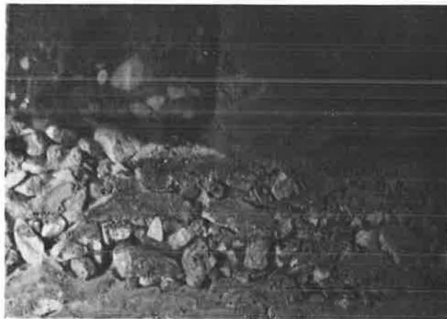
Figure 6. Fine material moving toward concrete slab and asphalt concrete shoulder joint in CA-9 base course.
