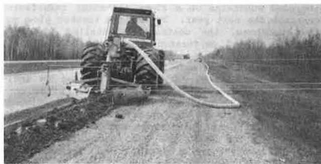
Figure 8. Trenchless plow mounted on rubber-tired tractor.
