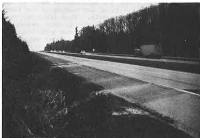
Figure 19. Water and fine material flowing out from beneath jointed concrete pavement on long gradient.
