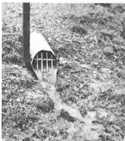
Figure 6. Discharge from pavement edge subdrain.
