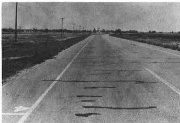
Figure 4. Transverse shrinkage cracking.
