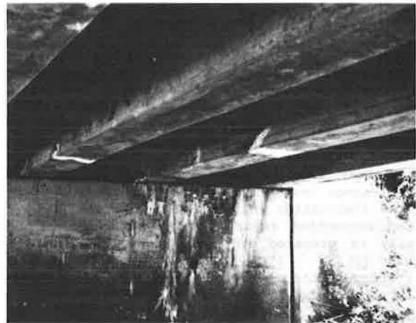
Figure 5. Condition of T-beams in bridge 2.
