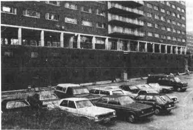
Figure 4. Partly constructed wall.
