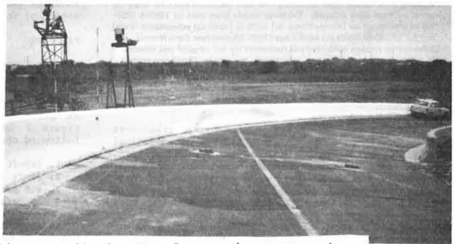
(b) Perpendicular New Jersey shape parapet
