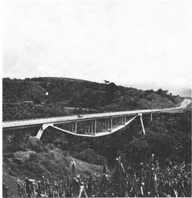
Figure 3. Rio Colorado Bridge.
