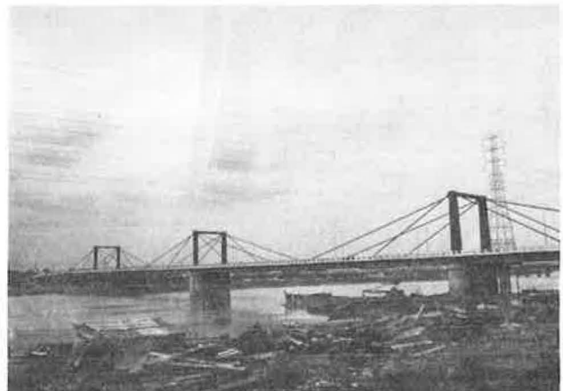
Figure 8. Kwong Fu Bridge.
