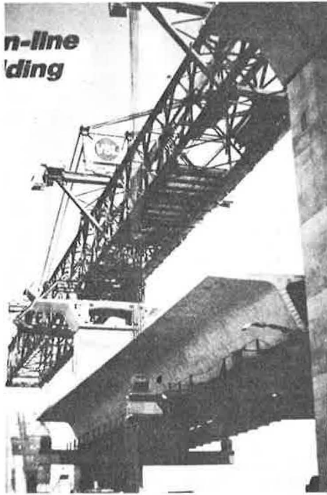
Figure 9. Long Key Bridge.
