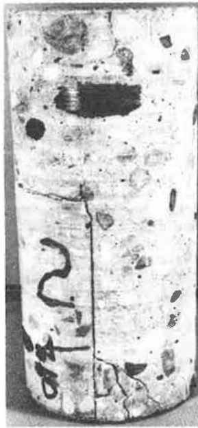
Figure 3. Core taken at center of panel over pier.
