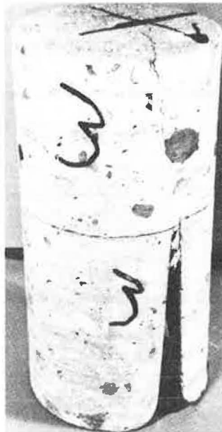
Figure 4. Core taken at quarter span over longitudinal joint.
