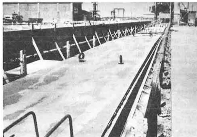
Figure 10. Knightstown deck was designed with built-in crown and with stirrups at ends of each slab to accommodate cast-in-place curb.
