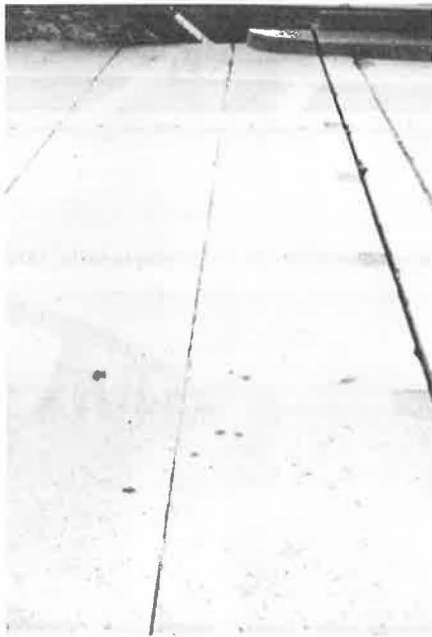
Figure 7. End element showing epoxy-mortar-filled blockouts as it appeared after 11 years of service.
