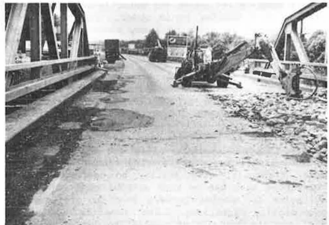
Figure 1. Old deck is broken up and dropped onto underlying creek bed.
