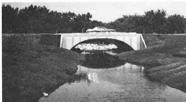
Figure 2. First BEBO arch built in the United States in Edina.
