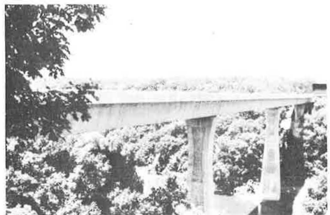
Figure 1. Kishwaukee River Bridge.
