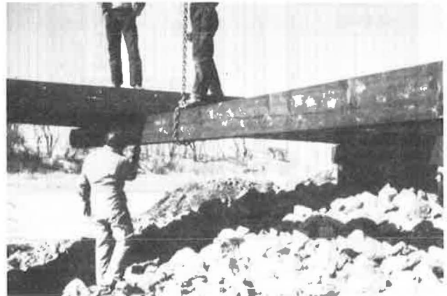
Figure 9. Installation of wood-spreader beam.
