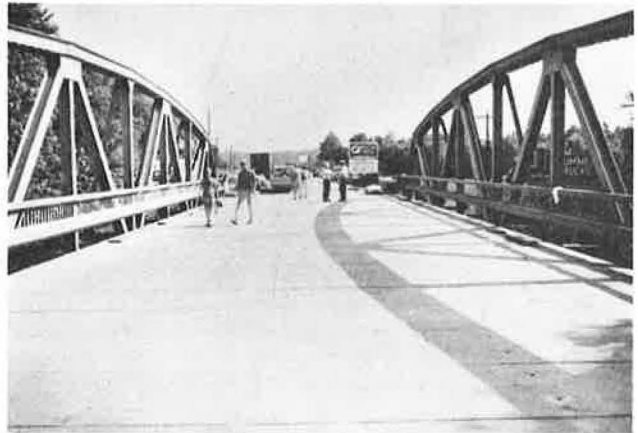
Figure 5. Completed deck near Bloomington prior to opening to traffic, 1970.
