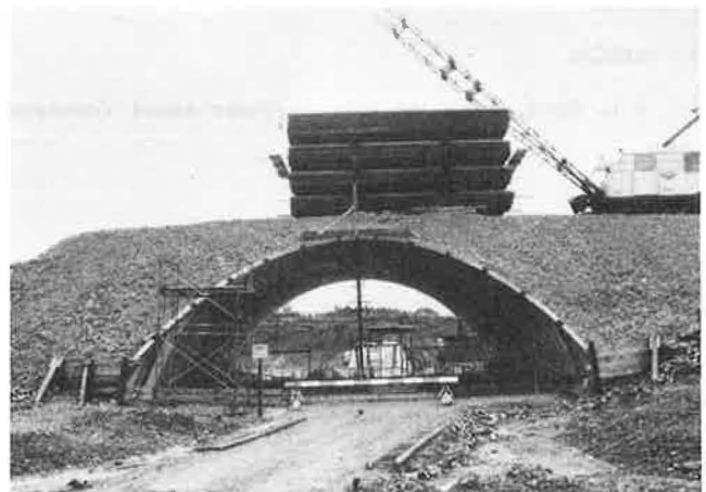
Figure 1. Original BEBO test structure in Zurich, Switzerland (1966).
