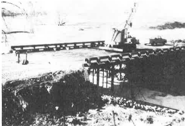
Figure 20. Completed timber bridge.
