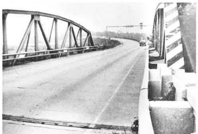
Figure 6. Precast deck near Bloomington after 11 years of service. No wearing surface or protective coating has been applied to deck. Rubber expansion joint shown here has performed well; however, southbound lane's joint has been damaged, probably by a snow plow.
