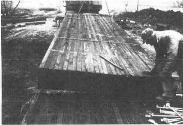
Figure 18. Panels are stockpiled at the job site.
