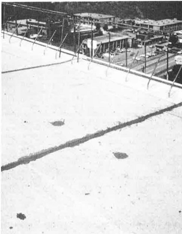
Figure 4. Placed modules were finished with cast-in-place parapet and latex-modified concrete wearing surface.
