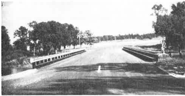
Figure 24. Example of treated-timber bridge.
