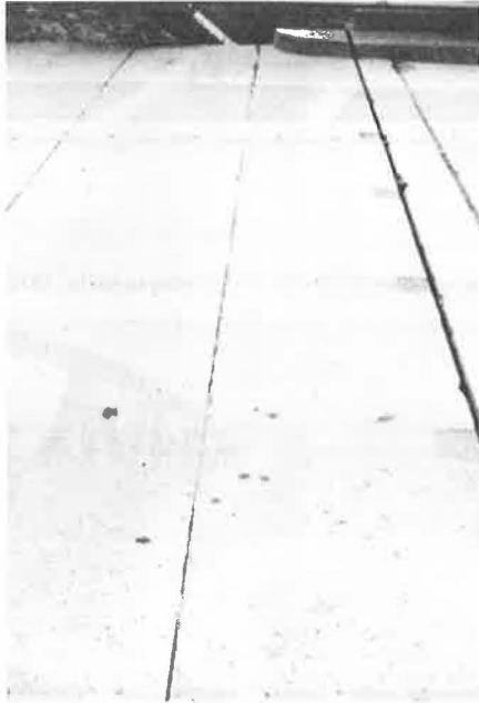
Figure 7. End element showing epoxy-mortar-filled blockouts as it appeared after 11 years of service.
