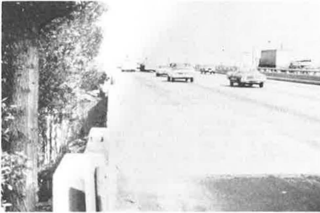
Figure 11. New deck is reopened to traffic during weekday peak period.
