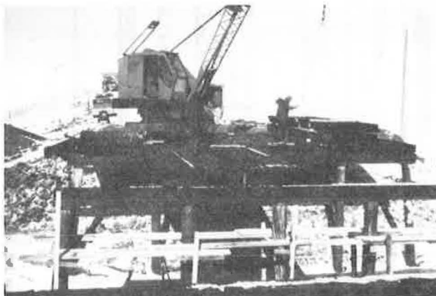
Figure 8. Support for deck panels.
