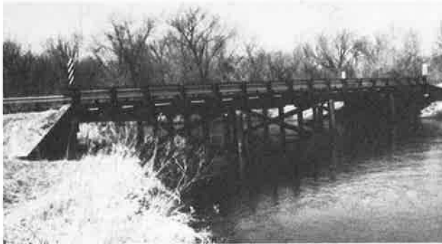
Figure 3. Example of timber bridge.
