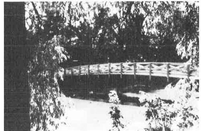
Figure 22. Timber bridge for pedestrians.
