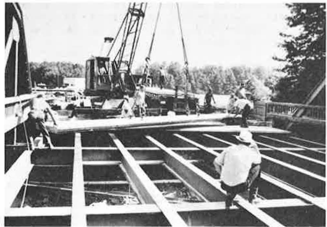
Figure 4. Precast, prestressed deck elements are positioned directly from delivery truck.
