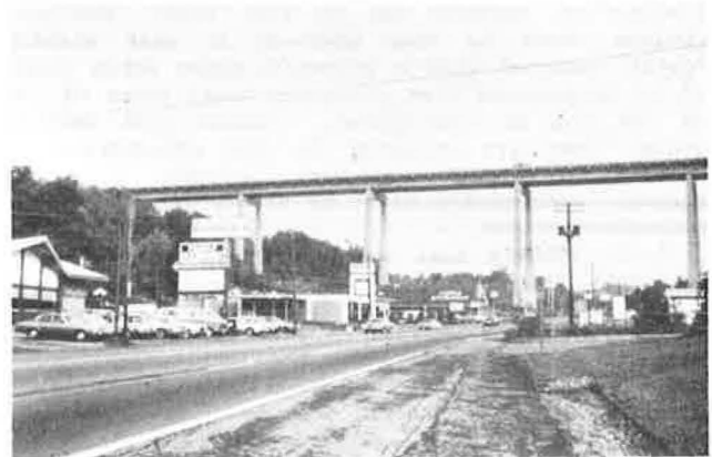
Figure 1. Pennsylvania Turnpike bridge.
