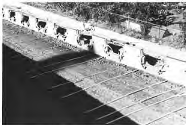
Figure 9. RE face panels held in position by wooden clamps with reinforcing strips attached.
