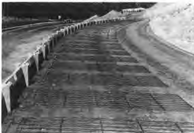
Figure 6. Steel bar mats for MSE in position on fill.
