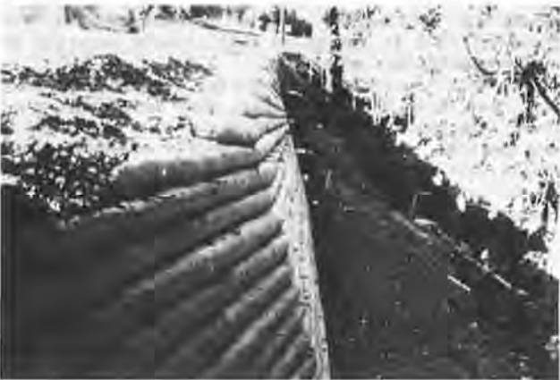
Figure 12. Bending wall to meeting existing slope.
