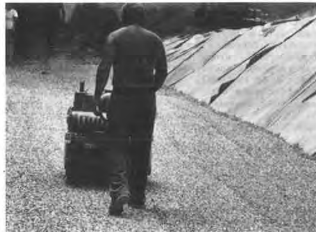
Figure 8. Compacting completed lift.
