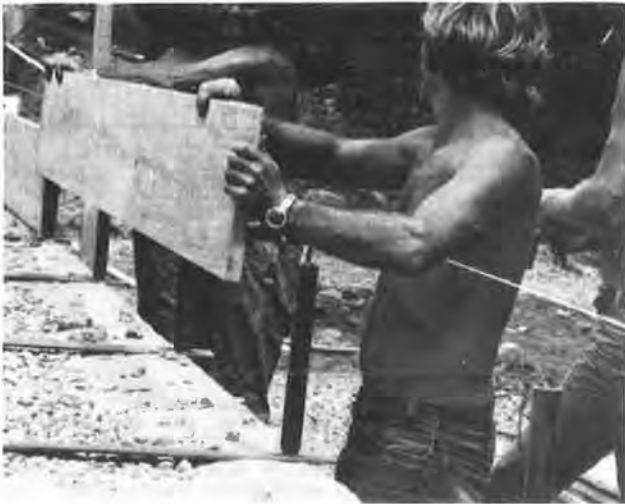
Figure 4. Placing temporary forms.
