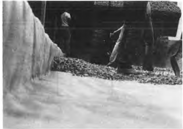
Figure 6. Forming berm for overlap.
