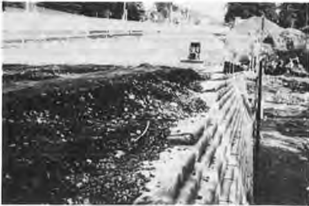
Figure 11. Stepping lifts to follow grade.
