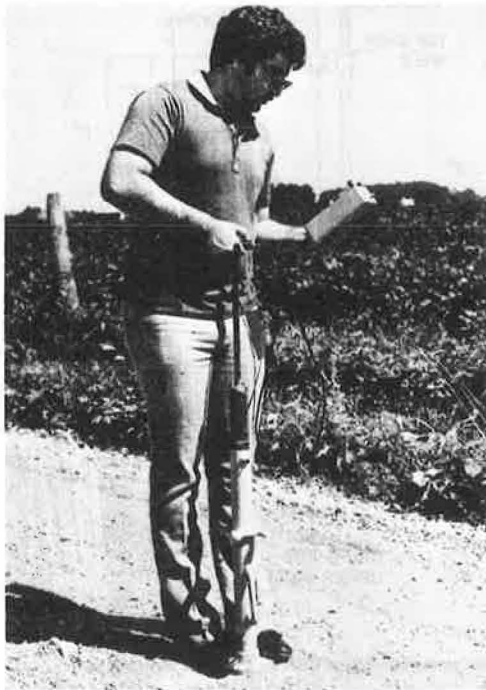
Figure 4. Clegg impact device.
