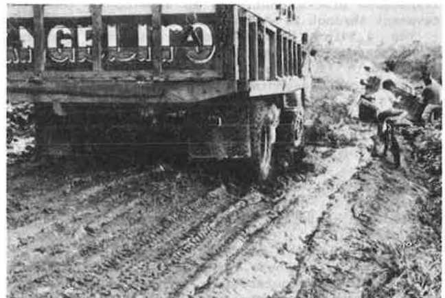
Figure 1. Failure of unsurfaced road.
