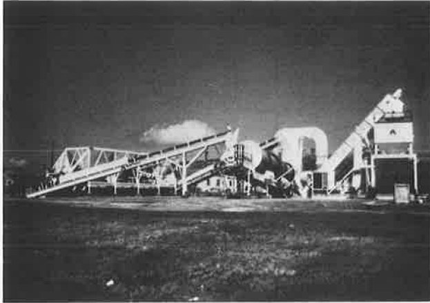
Figure 5. Drum mixer used at Lajes Air Force Base.
