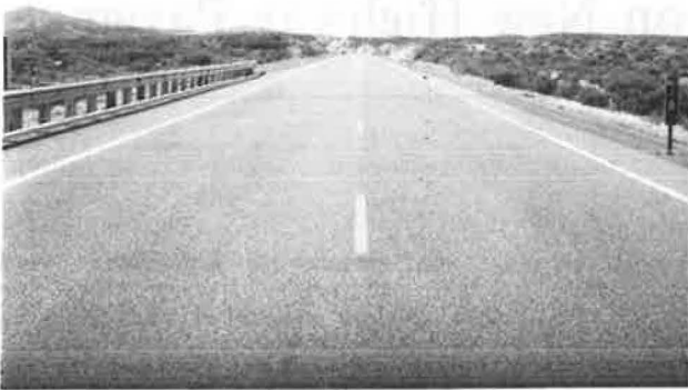
Figure 2. Test section 2: CTB, SAMI, and 1-in ACFC.
