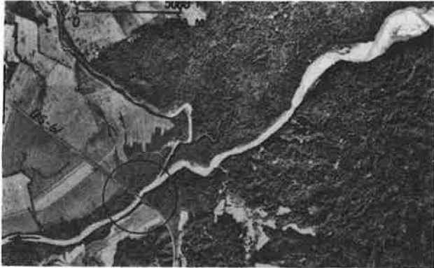
Figure 4. Degradation on Homochitto River at US-61 crossing near Doloroso, Mississippi, resulting in severe impact on lateral stability (indicated by change in stream form at right of photograph).
