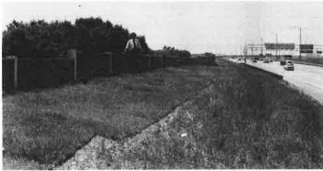
Figure 1. Steel noise barrier 1 m in height atop 3.7-m-high earth berm with 3:1 slope.
