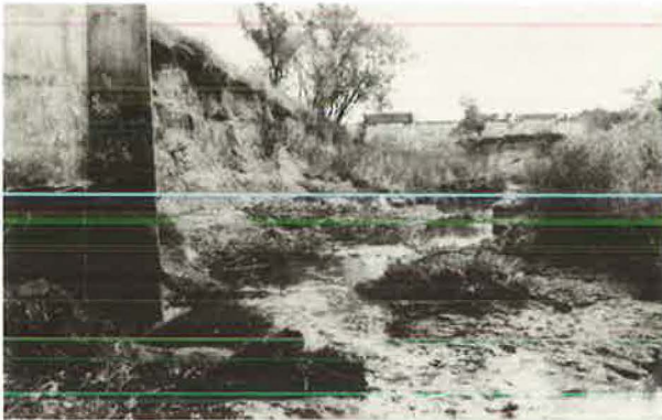
Figure 1. Degradation and resulting channel erosion at Middle Creek crossing of I-80 near Lincoln, Nebraska.
