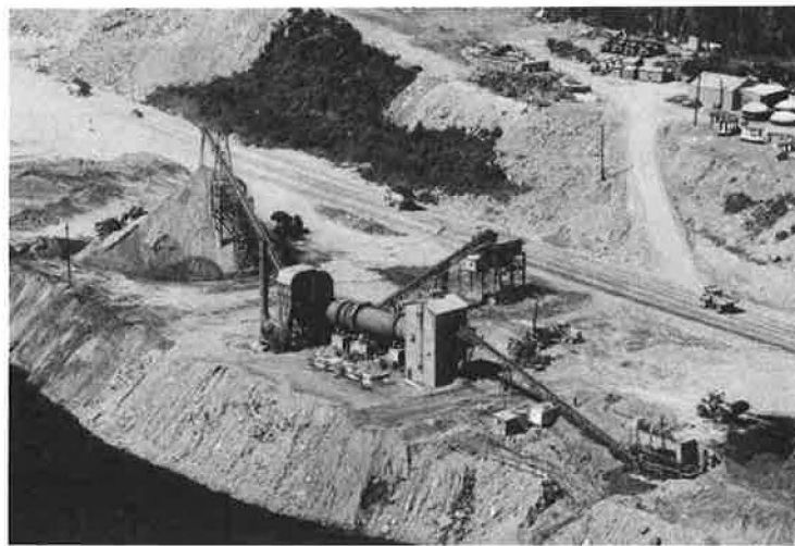
Figure 8. Rotary kiln drying plant.
