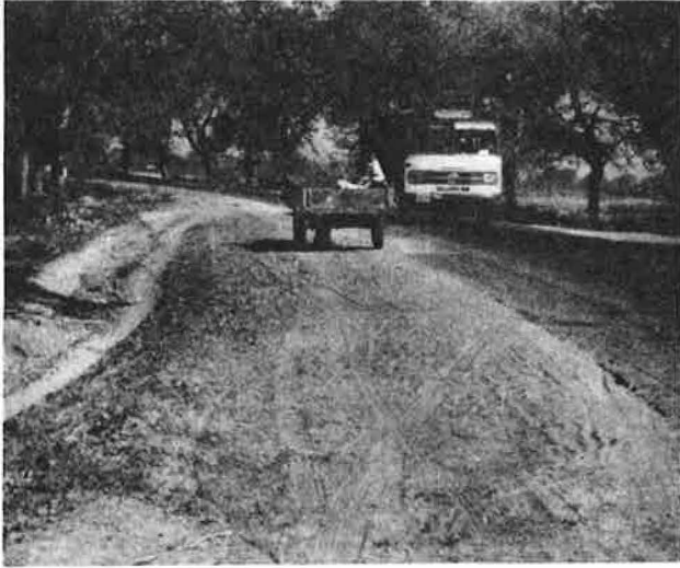
Figure 1. Single-lane road showing crossing between bus and bullock cart.
