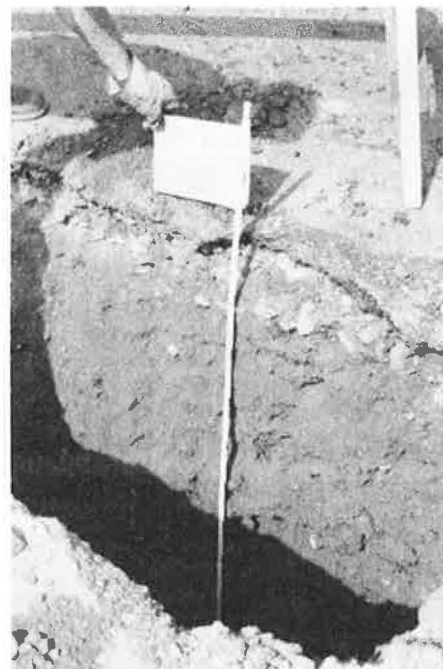
Figure 2. Typical pavement cross section.
