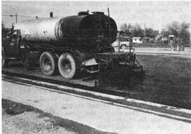
Figure 7. Placing of asphalt-rubber SAMI.
