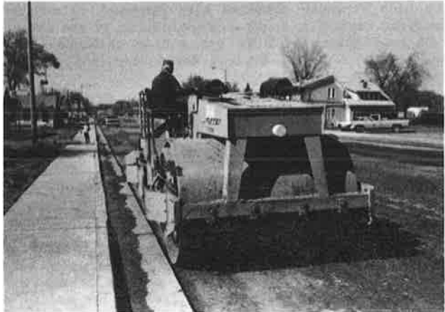
Figure 6. Finishing with pneumatic roller.
