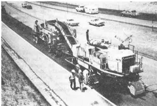
Figure 4. Cold planer feeding reclaimed material into towed screen and roll crusher.
