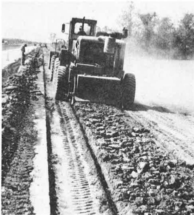
Figure 1. Chunk size of reclaimed asphalt-treated material after one pass of a hammermill.
