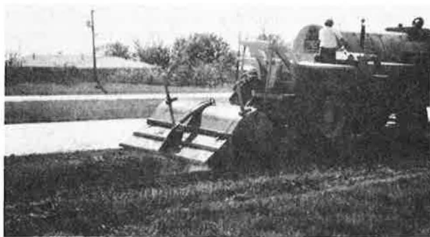
Figure 2. Pulvimixer adding asphalt binder to pulverized reclaimed material.
