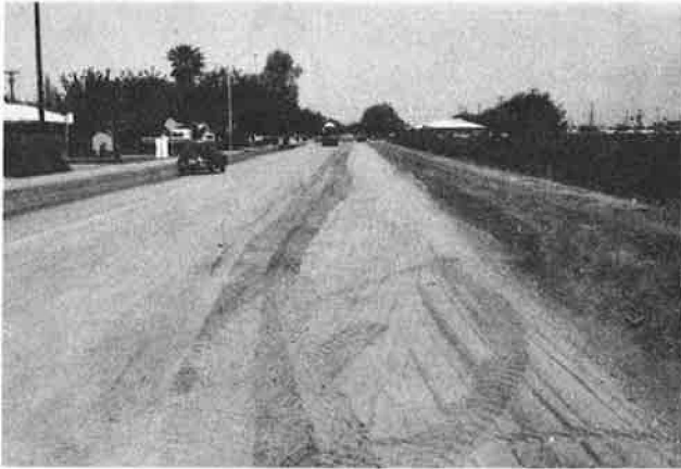
Figure 1. Grade preparation in alfalfa field soils on 55th Avenue, Phoenix, March 1971.
