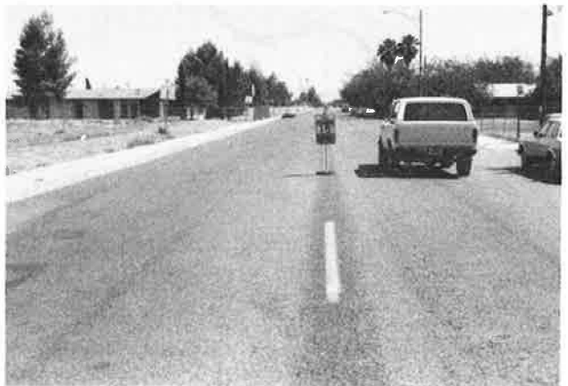
Figure 4. Surface condition in 1982 with only 0.5 in asphalt on native soil.
