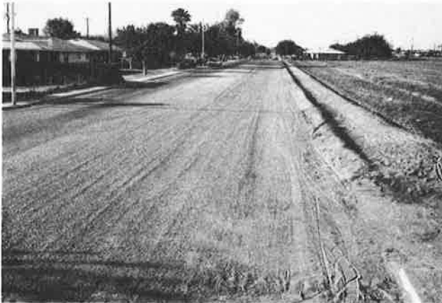
Figure 2. Completed surface immediately after construction with asphalt-rubber, March 1971.
