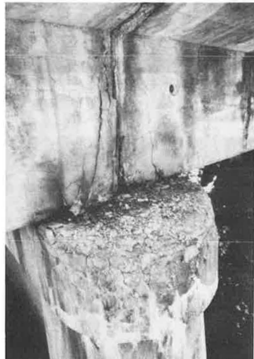
Figure 24. Cap damage.
