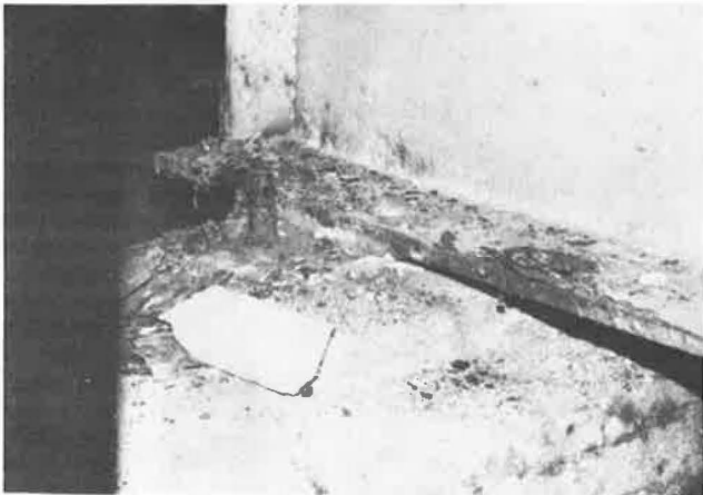
Figure 17. Bearing deterioration.
