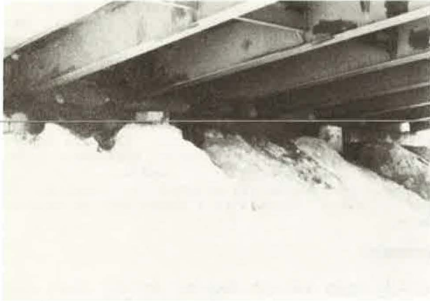
Figure 25. Embankment erosion.
