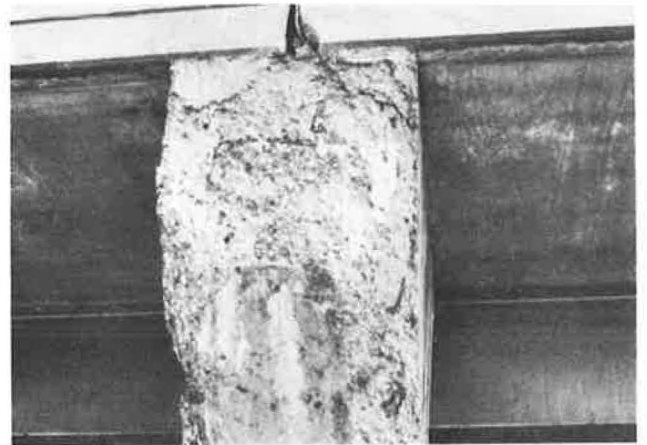
Figure 23. Cap damage.
