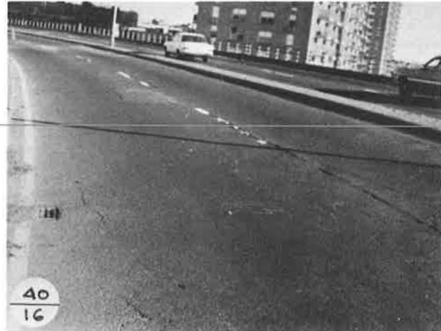
Figure 5. View of roadway.
