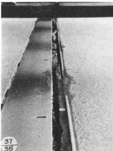
Figure 8. Deteriorated joint system.
