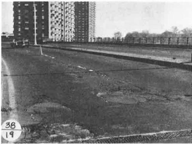
Figure 8. Deteriorated joint system.
