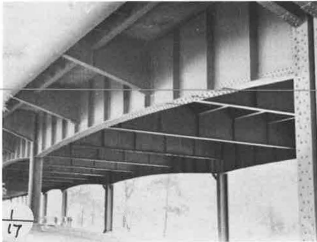
Figure 4. Structural steel bents.
