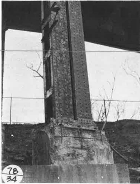
Figure 13. Deteriorated steel and concrete.
