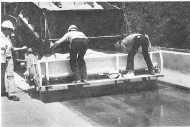
Figure 2. Silica aggregate is broadcast over resin.
