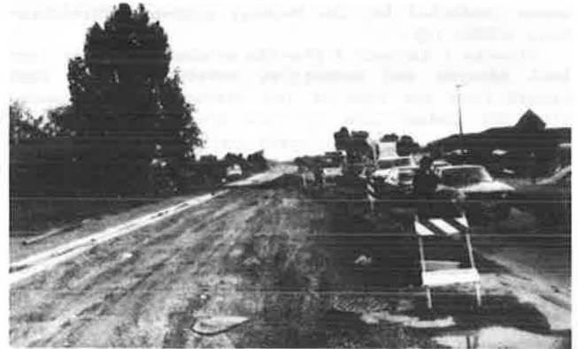
Figure 7. Absence of pedestrian access to abutting properties on highway widening project results in hazardous conditions.
