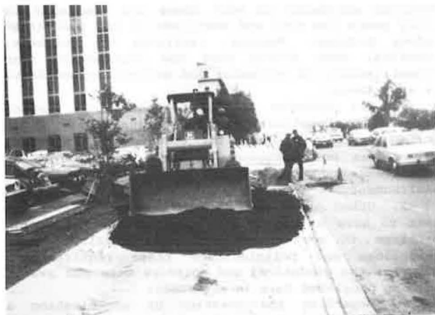
Figure 10. Example of bad pedestrian accommodation; pedestrian needs totally ignored on this side.
