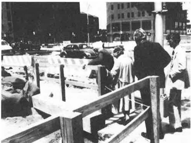
Figure 4. Temporary ramps with steep slopes create unsafe conditions for pedestrians with mobility problems.
