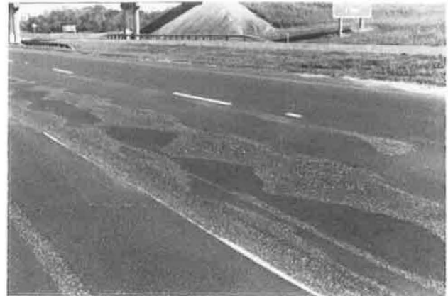
Figure 4. Planning that outlines the longitudinal variation in rutting and shoving distress.
