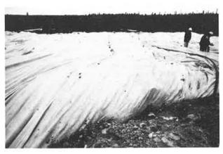
both sites. Significant lateral displacement of the peat was observed at the NBR-2 site. The difference in measurements between the settlement plates before and after construction indicated a lateral strain of the peat that varied from 20 to 80 percent. Heave of the peat at the toe and front of the advancing fill (Figure 13) was also observed and was on the
