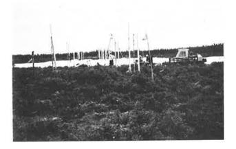
The test fills at NBR-2 were built to a height of 1 m above the muskeg surface. The final thicknesses varied from 2 to 3 m. The following is a description of the NBR-2 test fills.
