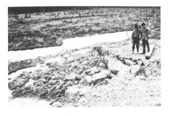
Figure 13. NBR-2, section B: lateral displacement and heave of peat.
