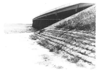
stability of the sand-cement constructed facilities, as shown in Figures 12 and 13. No erosion problems were apparent at any of the drains, slopes, and seawalls protected by the sand-cement armoring system, which indicated that the installation was functioning as designed. The armoring, in most cases, has held up completely. Some surface wear was noticeable; however, no washouts of the rip-rap were observed.
