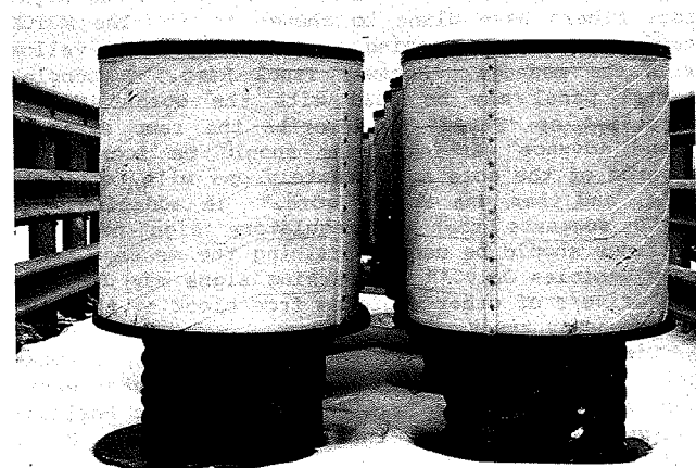
Figure 5. Sand-barrel impact attenuators on pedestals at end of the truck escape ramp on NY-28 in New York.
