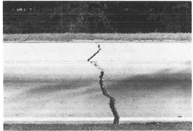
Figure 4. Bituminous patch in existing CRCP.
