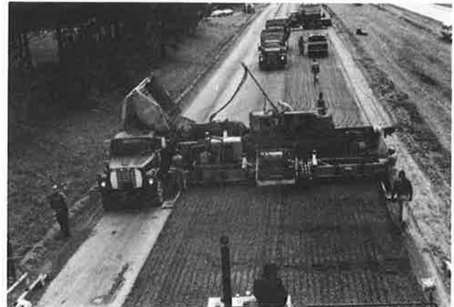
Figure 11. Rear view of concrete spreader.
