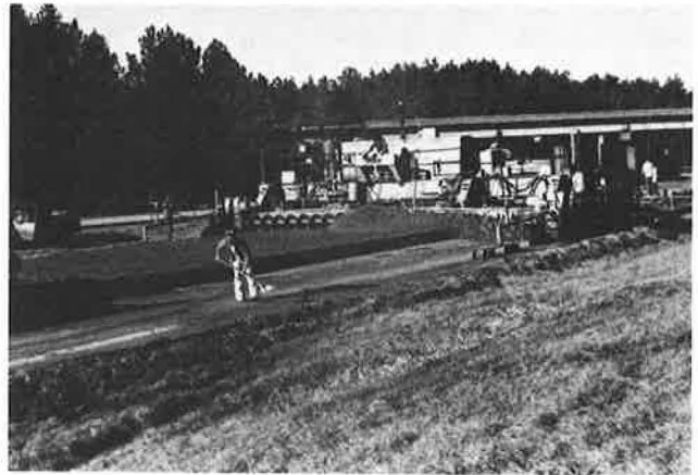
Figure 12. Front view of concrete paver.
