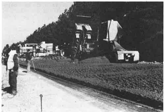
Figure 13. Placing additional concrete on outside lane and shoulder.
