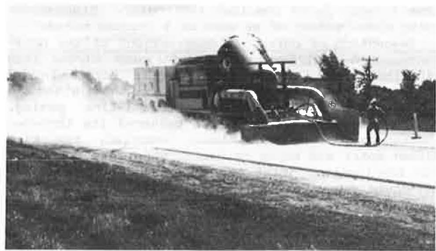
Figure 2. Pavement sandblasting machine in operation.
