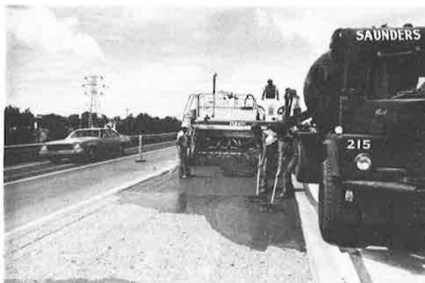
Figure 3. Middle-lane grouting and paving adjacent to previously overlaid median lane.
