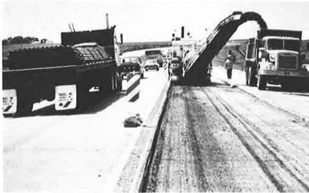
Figure 6. Milling asphaltic concrete 10 in. deep and 12.5 ft wide.
