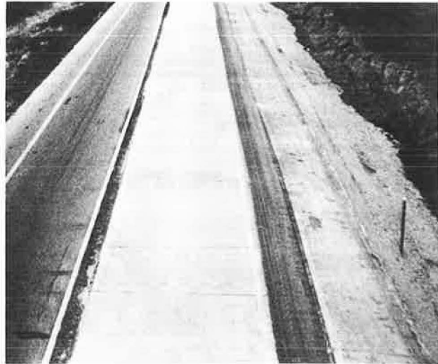
Figure 9. Finished portland-cement concrete inlay.
