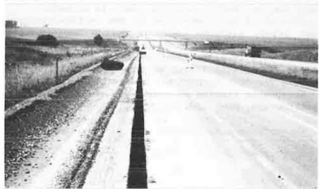
Figure 4. Trenching 42 in. deep for placement of longitudinal drain.
