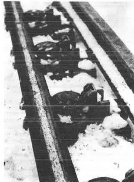
Figure 11. Prototype hold-down latches, Seinajoki Yard.
