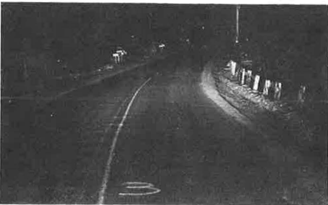
Figure 6. White premixed paint (centerline, upper left) after 12 years of service; rest of line painted over in yellow.
