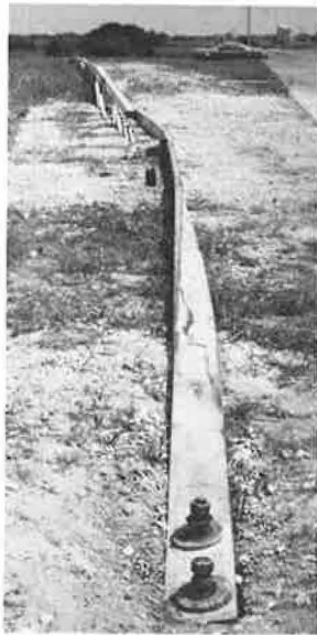
Figure 6. Rail after test 6.
