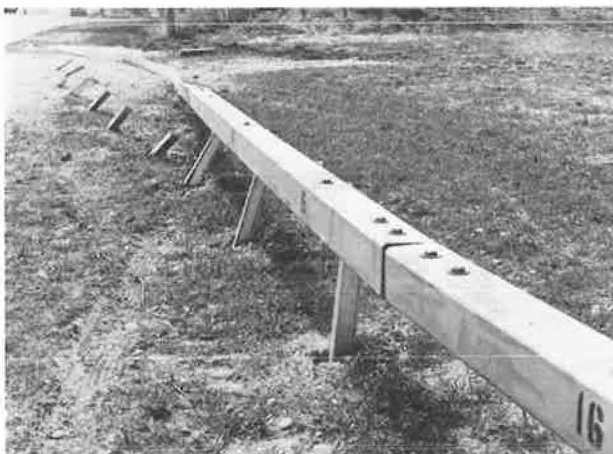
Figure 4. Rail damage after test 4.
