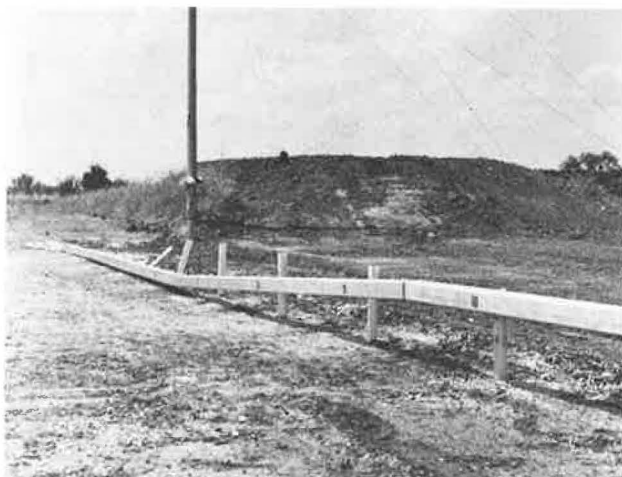
Figure 2. Rail after test 1.
