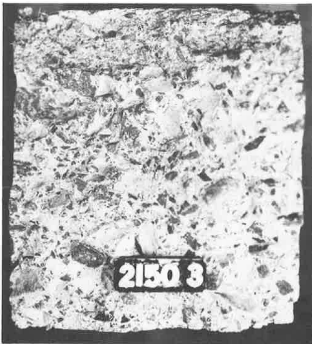
FIGURE 11 RCC topped with FRC (close up view).
