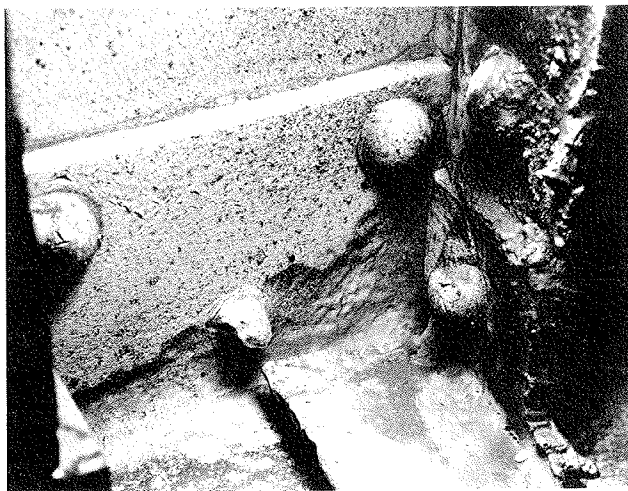
FIGURE 6 Preexisting crack in compression flange next to bracing connections.
