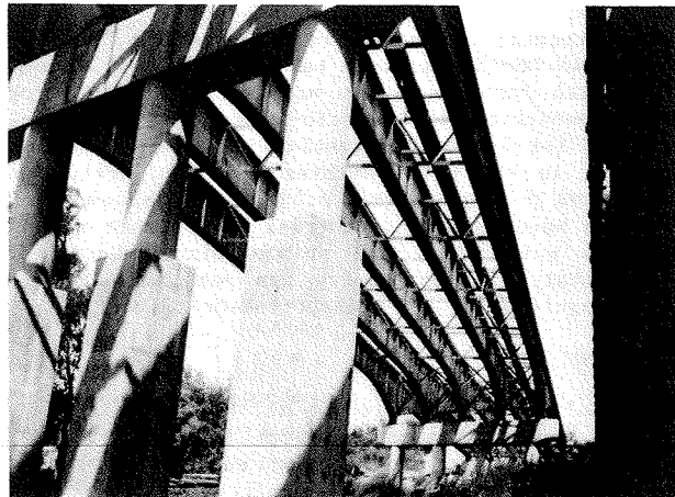
FIGURE 3 Fifth Street Bridge, Lynchburg, Virginia (under construction).
