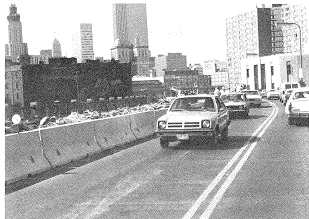
FIGURE 7 Traffic barrier on upstream half of bridge.
