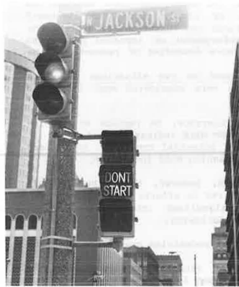
FIGURE 2 Devices tested to indicate the clearance interval: symbolic pedestrian signal explanation sign (left) and DONT START signal display (right).
