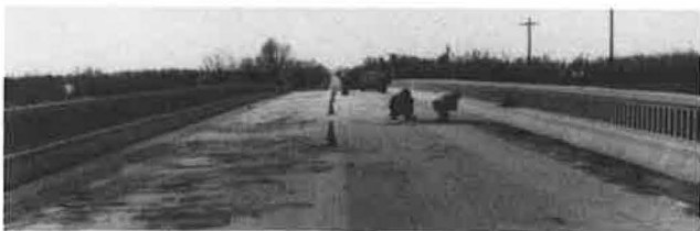
FIGURE 1 A 16-year-old polypropylene fabric membrane covering part of the deck in right foreground.
