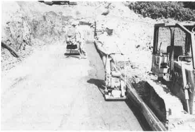
FIGURE 11 Compacting class-B backfill near the forms.
