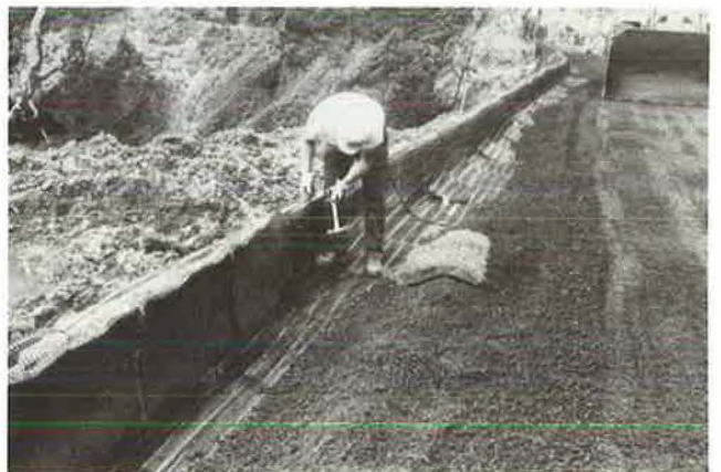
FIGURE 10 Hanging sod on back of forms.
