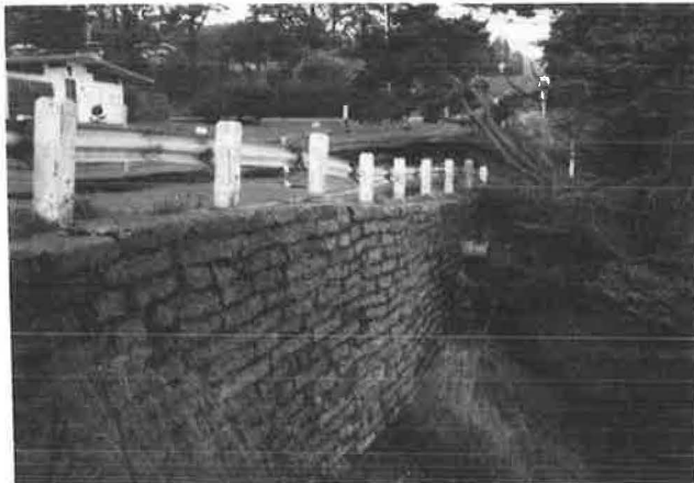
FIGURE 2 Site before construction.
