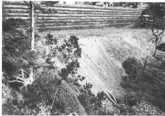
FIGURE 14 Completed geogrid wall.
