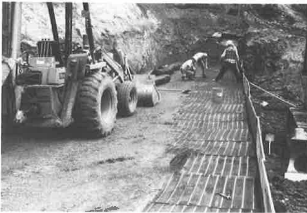
FIGURE 12 Pinning geogrid overlap in place.
