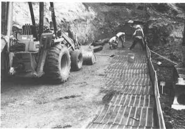
FIGURE 12 Pinning geogrid overlap in place.
