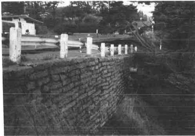
FIGURE 2 Site before construction.
