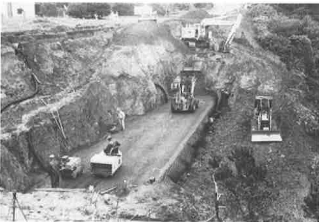
FIGURE 13 General view of construction site during backfill compaction.
