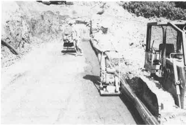
FIGURE 11 Compacting class-B backfill near the forms.
