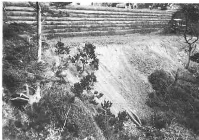
FIGURE 14 Completed geogrid wall.
