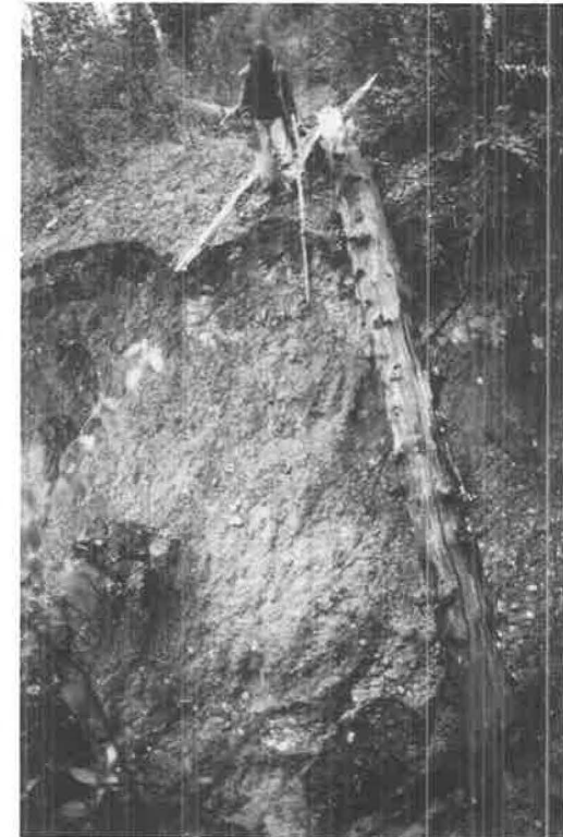
FIGURE 7 Scarp at drill hole 1 after 1982 failure of Cable Car landslide.
