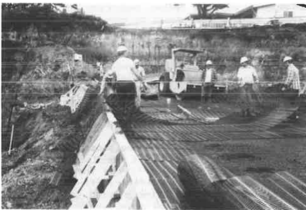
FIGURE 16 Modified forming system and heavy vibrating roller used for backfill compaction.
