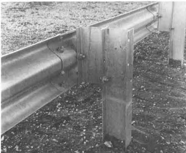
FIGURE 2 G4(1S) barrier installed on 6:1 slope.
