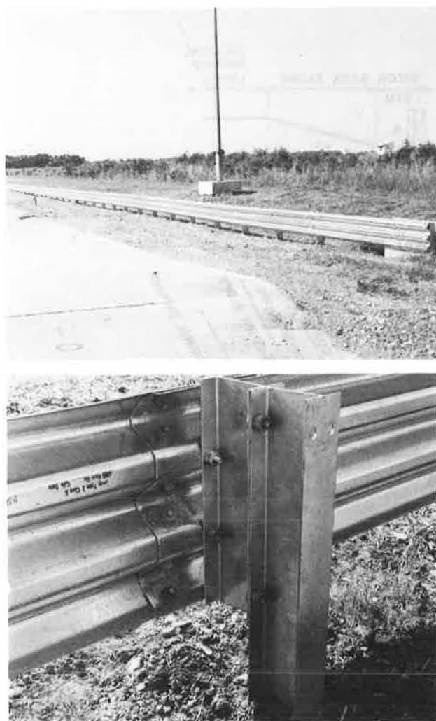
FIGURE 4 G9 barrier installed on 6:1 slope.
