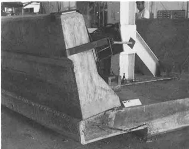
FIGURE 7 Typical crack patterns for Texas T5 concrete post and bridge deck.
